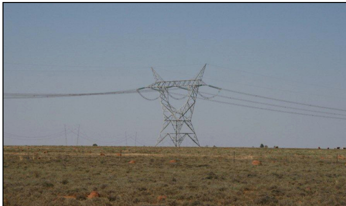
Figure 8.6: Photo showing the highly visible nature of a powerline
